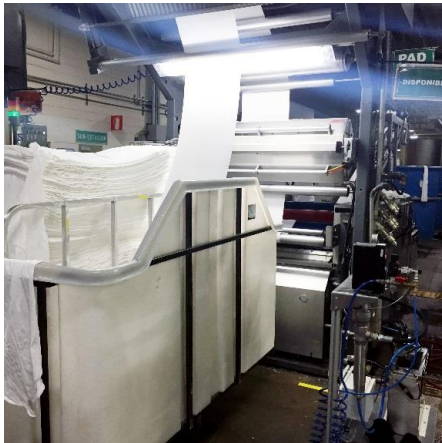
Baldwin's Precision Application System at HanesBrands.
